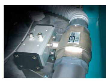
**AVC** is an automatic ventilation closing system which allows, in the event of radioactive substance release via hot cell ventilation conduits, to block ventilation, close the inlet conduit and the air outlet of the hot cell and simultaneously open the valve connecting the hot cell to the contaminated air storage system (see Comecer ACS).
